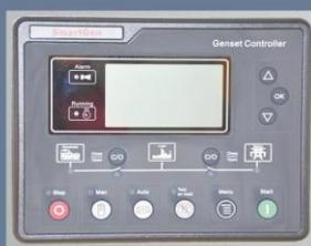
The control panel will show the temperature for water/oil, speed, frequency, voltage, current, malfunction.
